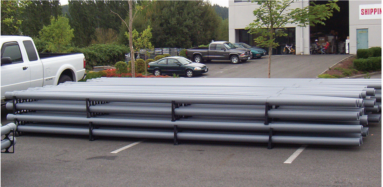
Photo 2. These partially assembled conduit duct banks, prepared at the SASCO Electric prefabrication warehouse, not only reduce field installation time, but help cut down on excess packaging making its way on a LEED project site.
