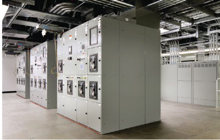
Figure 2: The design of this 7th-floor data center, handled by engineers from AlfaTech Consulting Engineers, includes a built-up cooling system. Courtesy: AlfaTech Consulting Engineers
