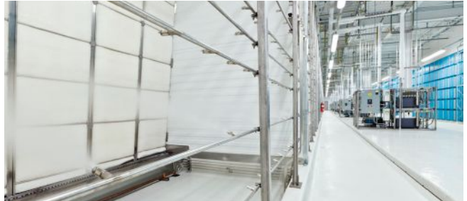
Figure 3: This data center in Prineville, Ore., features a mechanical air-handling system with evaporative cooling pumps and spray nozzles. Courtesy: AlfaTech Consulting Engineers
